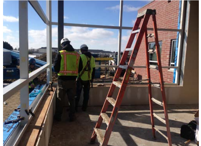
6. Strength Training: Crew installing large corner window.
