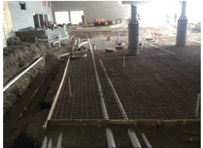
4. Rec. Pool: Rebar and formwork for waterslide plunge area.
