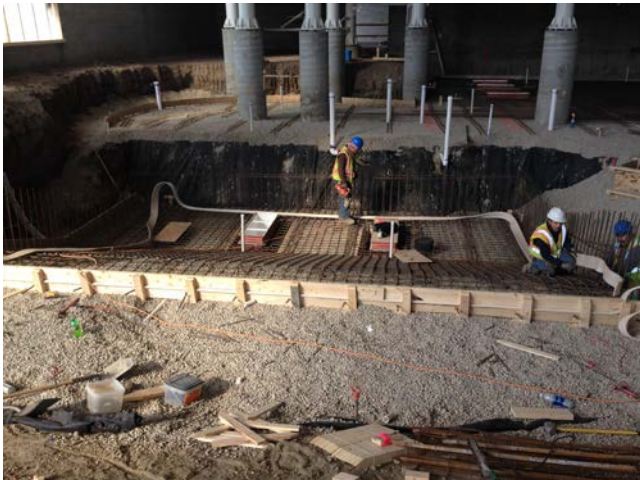
3. Rec. Pool: Rebar and formwork for deep end pool bottom.
