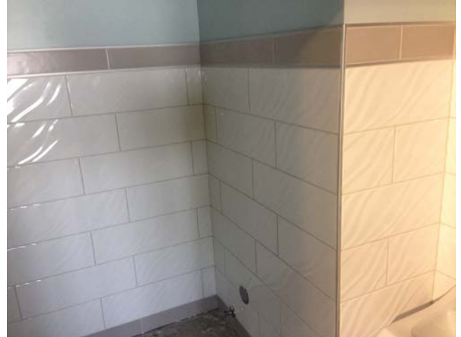
2. Childcare Toilet: Tilework complete and grouted.
