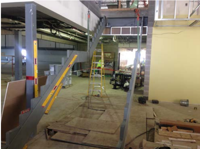
5. Lobby: Grand stair installation is underway.
