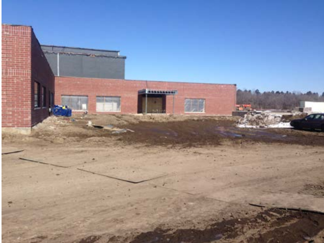
1. Connecting Link: Masons have completed exterior brick.
