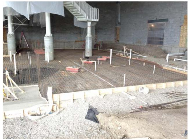
4. Rec. Pool: Rebar and formwork ready for pour next week.
