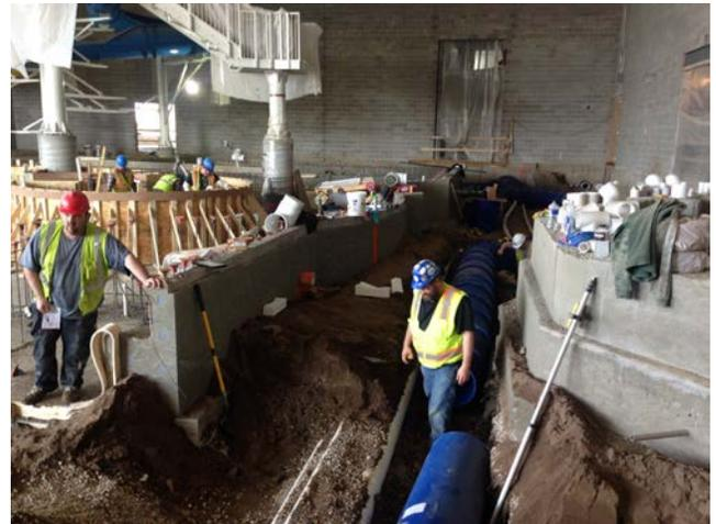
4. Rec. Pool: Crews working on forms & underground duct.
