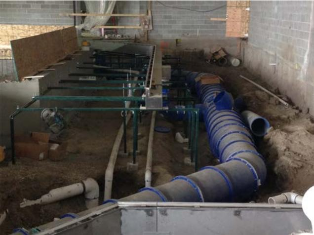
5. Rec. Pool: Ductwork and trench drains are installed.
