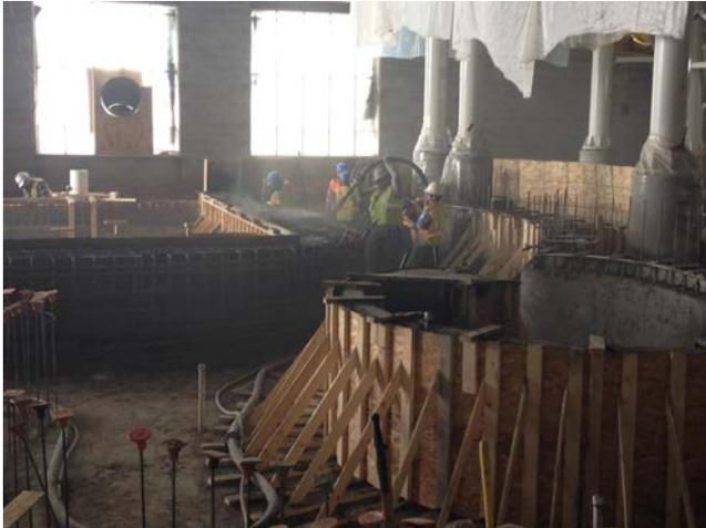
4. Rec. Pool: Crews working on pouring concrete walls.
