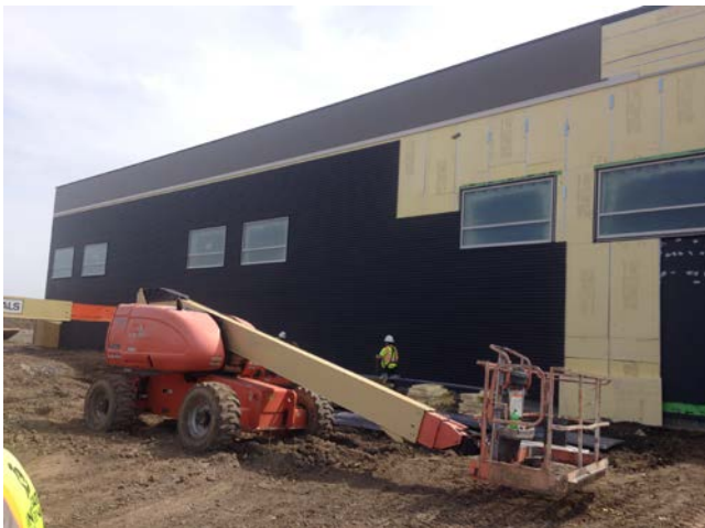
5. North Exterior: Metal panel installation is nearly complete.
