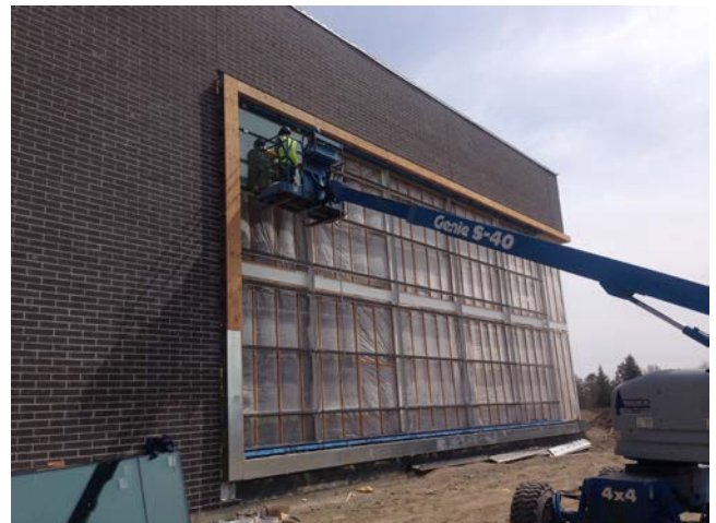
6. West Exterior: Glass installation at recreation pool.
