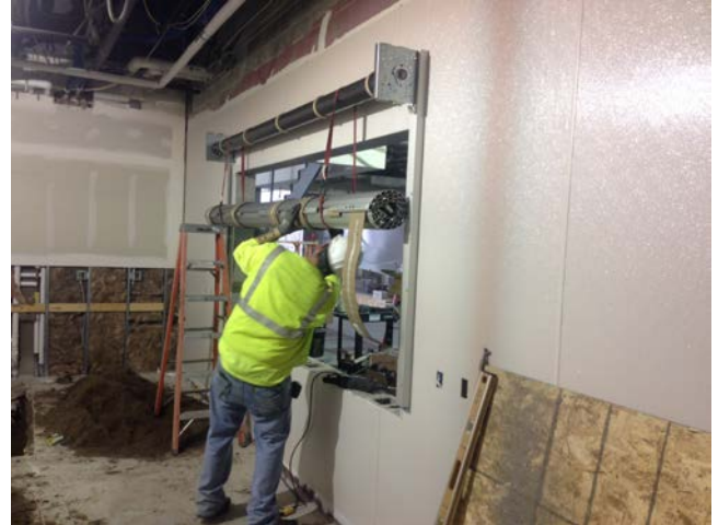
2. Kitchen: Coiling door install is underway.
