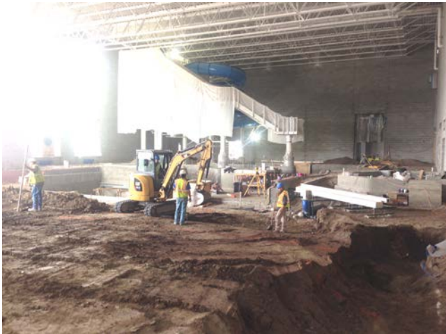
3. Rec. Pool: Excavation for phase II is underway.
