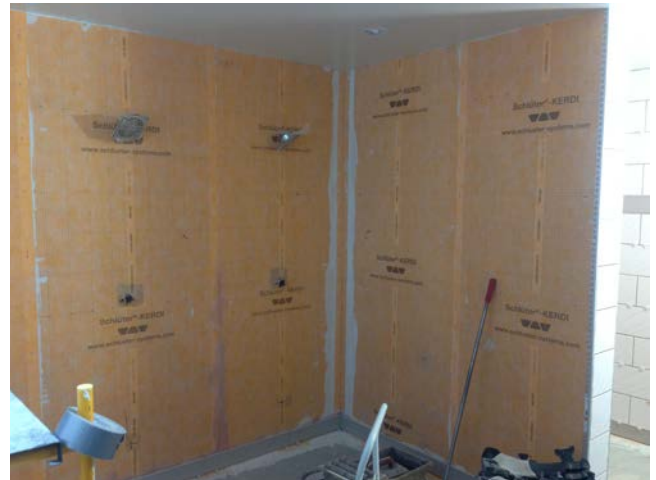
4. Showers: Waterproofing behind tile is installed.
