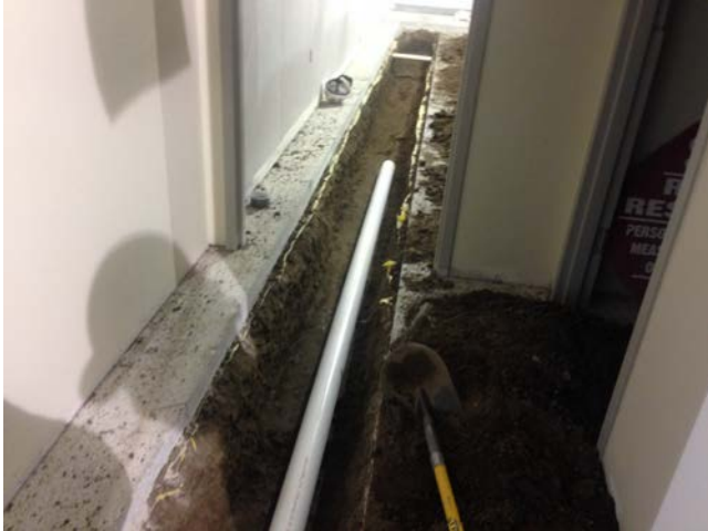
1. Kitchen: Piping for kitchen sink is being installed.
