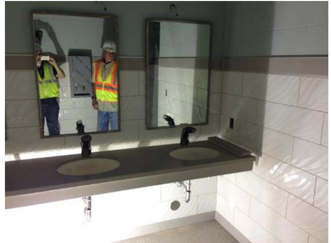
2. Toilet Rooms: Counters are installed & plumbing installed.
